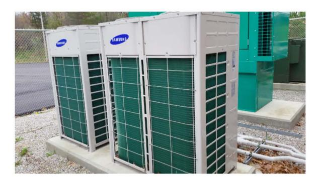
The main system uses a 28-ton condensing unit with a mix of four-way cassette and ducted units ranging from a half ton up to four tons. This system serves the entire building. The second, 14-ton system provides redundancy for critical areas of the building.
