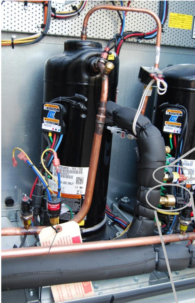
Figure 151 - Digital Compressor Circuit
