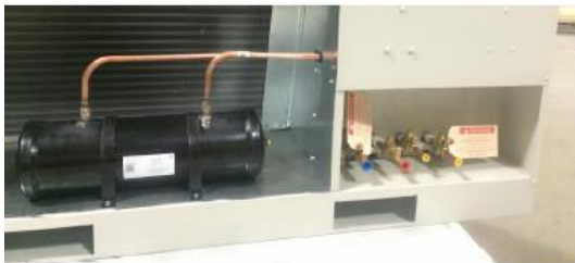
Figure 100 - Horizontal Receiver Installed in Condensing Unit
