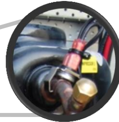
Figure 148 - Digital Discharge Thermistor
