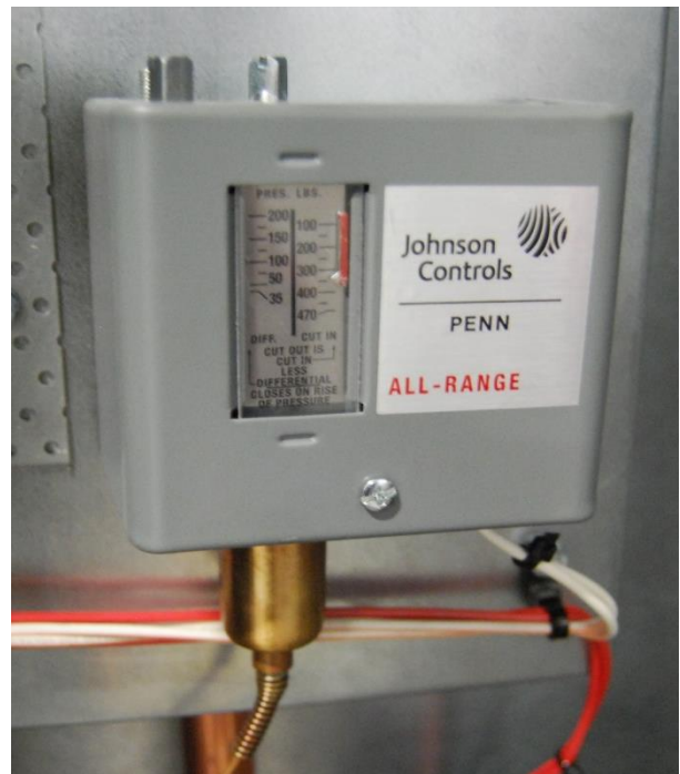
Figure 136 - Adjustable Fan Cycling Switch
