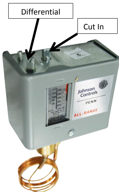
Figure 137 - Adjustable Fan Cycling Switch - Split Systems
