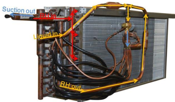
Figure 67 - Reheat Coil in AHU
