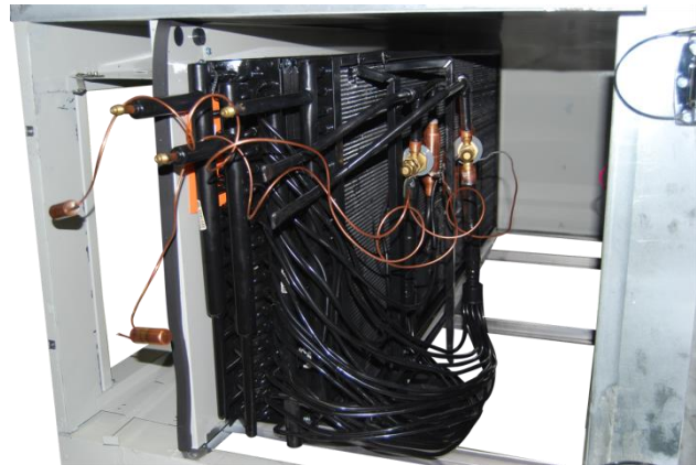
Figure 47 - E-coated DX Coil
