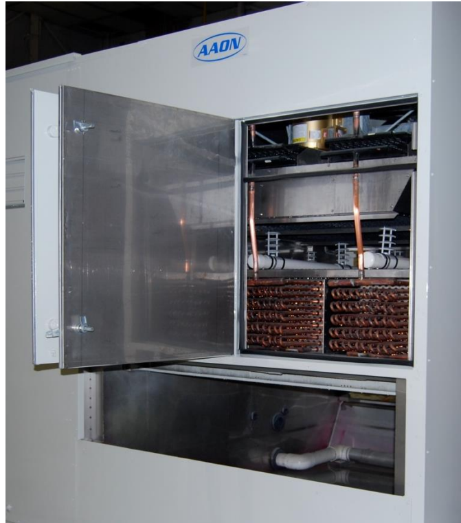
Figure 54 - Evaporative-Cooled Condenser
