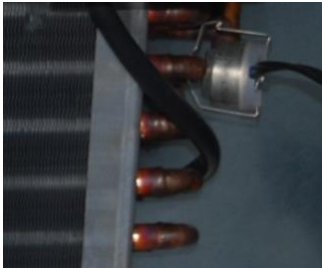
Figure 81 - Freeze-Stat
