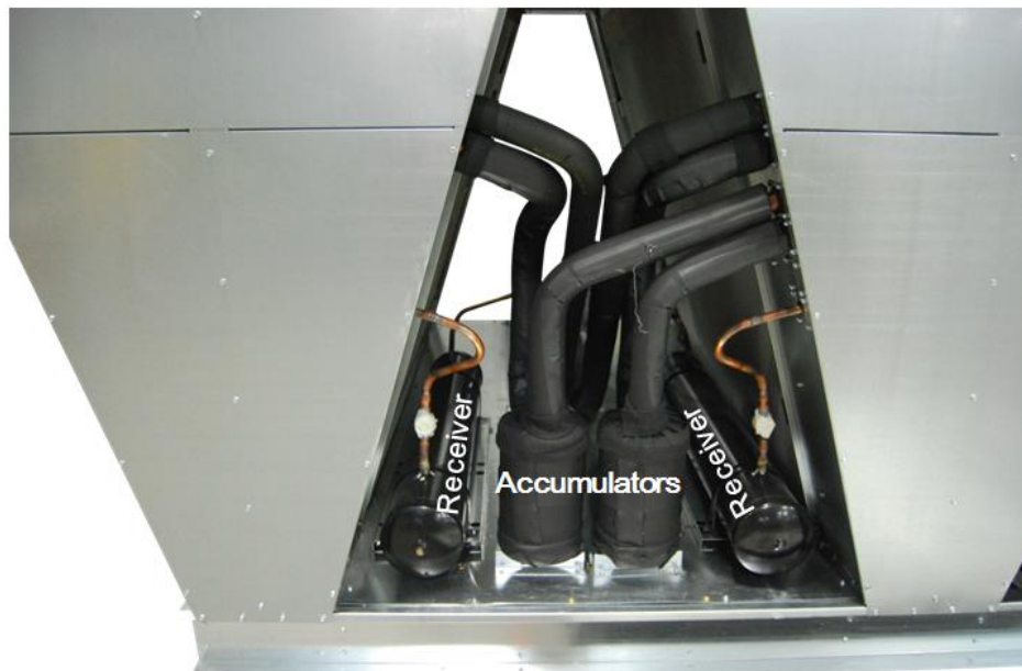
Figure 105 - Suction Line Accumulators & Liquid Line Receivers Installed in a Heat Pump Condensing Unit
