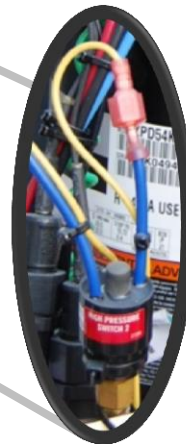
Figure 149 - High Pressure Switch
