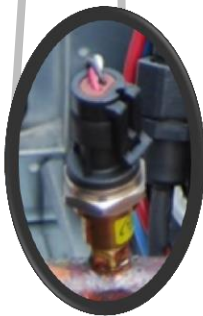
Figure 150 - Discharge Pressure Transducer
