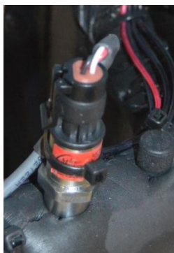
Figure 39 - Suction Line Sensors
