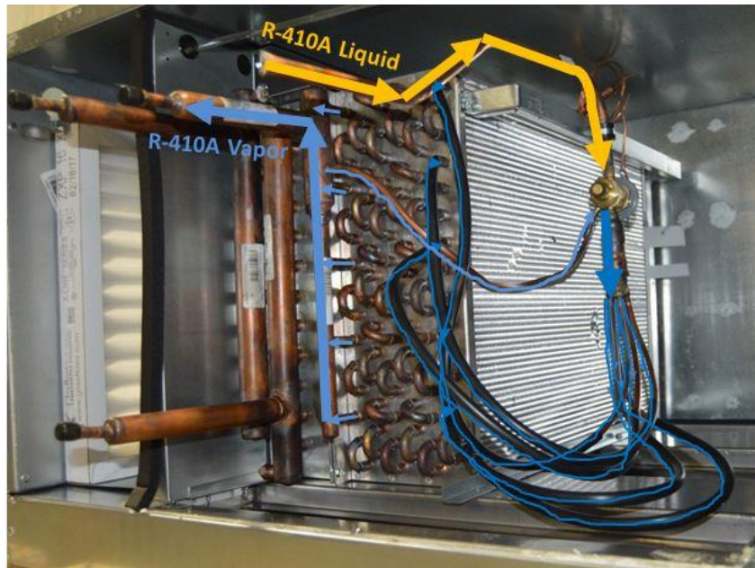
Figure 44 - Refrigerant Flow through a DX Coil
