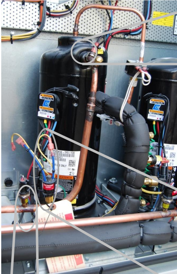
Figure 147 - Digital Compressor Circuit
