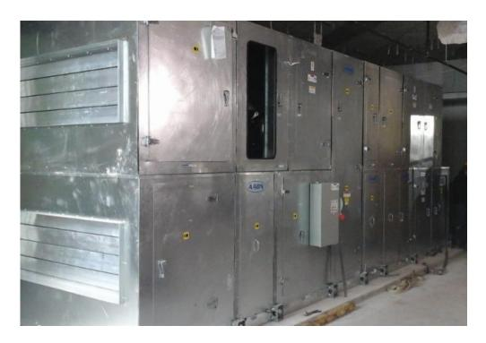
5 AAON Water Cooled Dedicated Outdoor Air Systems were needed to accommodate the buildings HVAC needs. These systems work great when you need temperature and humidity control in large areas. They make use of 100% outdoor air, and then adjust humidity and temperature based on the climate of the room. Not only is this efficient, but
