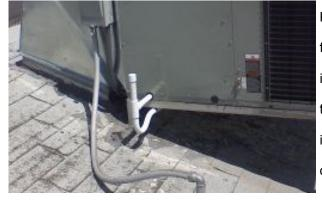
Keep the drain dry and protected in the winter to prevent freezing and check to be sure it is connected properly during the inspection as it may have fallen off during the winter months. If this is not check and cleaned out properly it could cause a lot of water damage in the space below due to the condensate pan overflowing.
